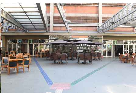
Main entrance Convenience Area
